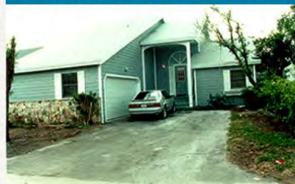
Level 2 - Major damage; habitable
